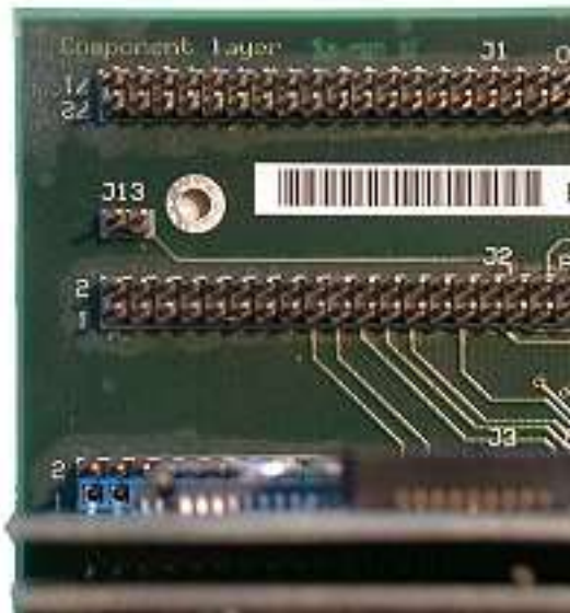
Figure 58. A close-up of the reset jumper in section 1.
